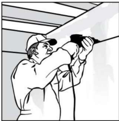
1. Fixing the perimeter L-<-hannel
