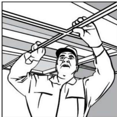
3. Installing the suspended grid
